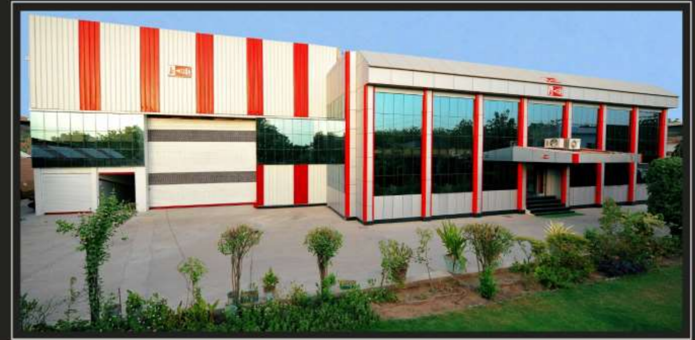
HEAD OFFICE, JODHPUR, INDIA
